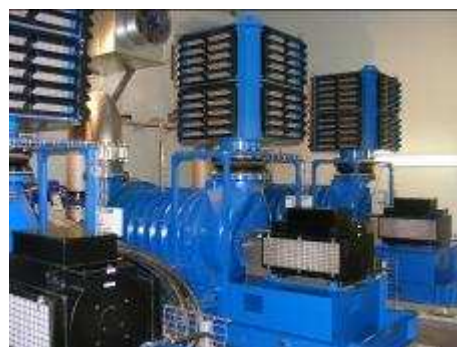
V-CENTRIF: Brive La Gaillarde Waste water treatment
